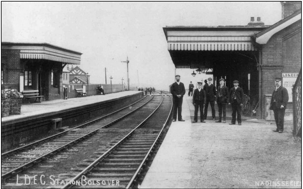
Bolsover Station in LD&ECR days looking west towards Chesterfield. The photographer is stood under the footbridge at the east end of the station. The occupation crossing can be seen just beyond the platform ends.
