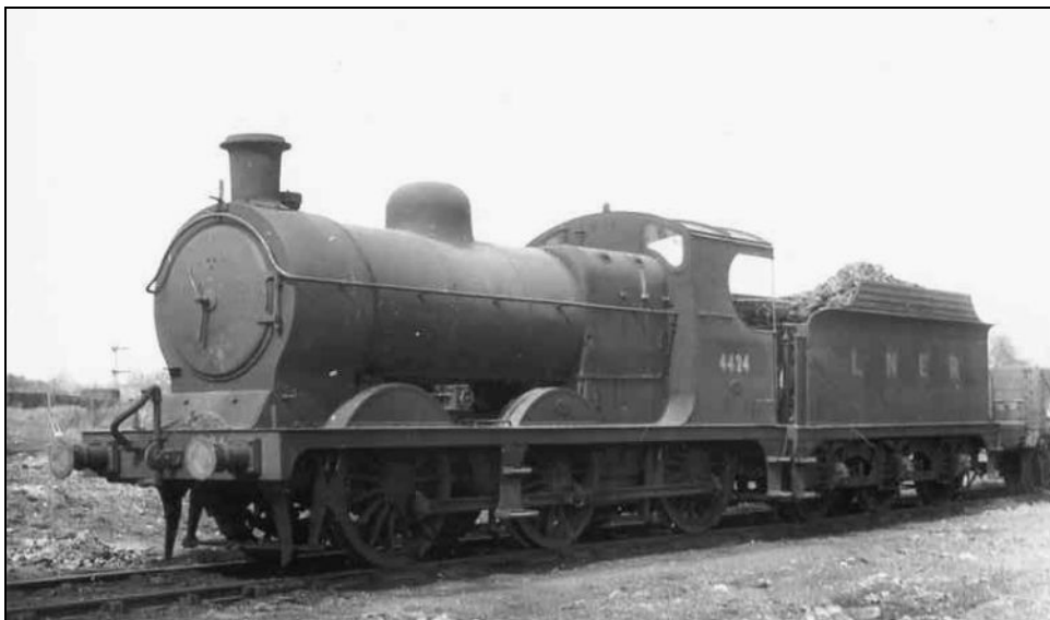
LNER class J11 0-6-0 no. 4424 (1946 numbering). This class was a development of Robinson's first 0-6-0 design (LNER class J10). It became the standard small goods engine for the GC with 174 being built over the period 1901-1910 in numerous batches from different manufacturers. Known as the 'Pom-Poms' because their noisy bark sounded like the rapid firing gun of that name used in the Boer War. Some of the class were later fitted with piston valves and designated J11/3. No. 4424 retained its slide valves until withdrawn in 1958.
