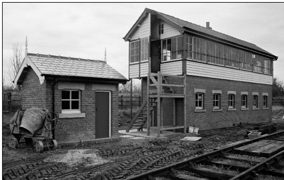
The former Neasden South Junction box on its new brick base at the Nottingham Transport Heritage Centre at Ruddington. Renovation is well advanced. Alongside is the newly built lamp room.
