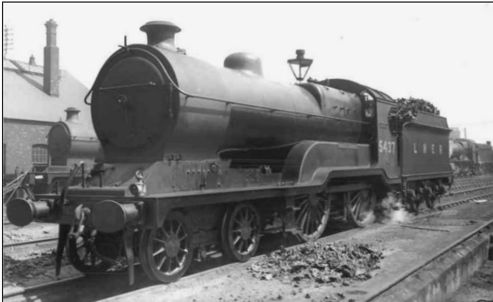
LNER class D10 4-4-0 no. 5437 Prince George. Robinson's second 4-4-0 design was introduced in 1913 and they were all originally named after directors of the GCR, hence the class was known as the 'Directors'. No. 5437 was originally named Charles Stuart Wortley before being renamed Prince George in 1920. The success of the class led to the introduction of a further batch of 'Improved Directors' (LNER class D11) from 1919. The most noticeable distinguishing feature between the two classes is the cab style - cut-out cabs on the D10s and window cabs on the D11s. No. 5437 survived until 1955 as no. 62658.
