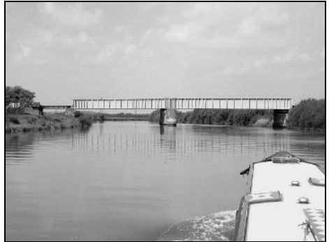
The railway bridge over the River Trent at Gainsborough.
